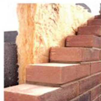
Brick wall with insulation
